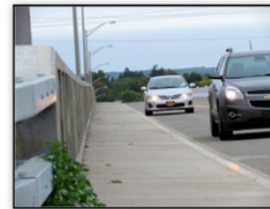
Above: only a curb now for protection Below: before the rehab, guardrails, guiderails, and bike safety fences
