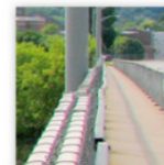
Above: only a curb now for protection Below: before the rehab, guardrails, guiderails, and bike safety fences
